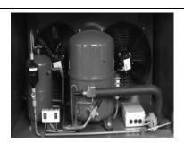
REFRIGERATON: Mechanical single stage refrigeration system with hermetic compressor.
